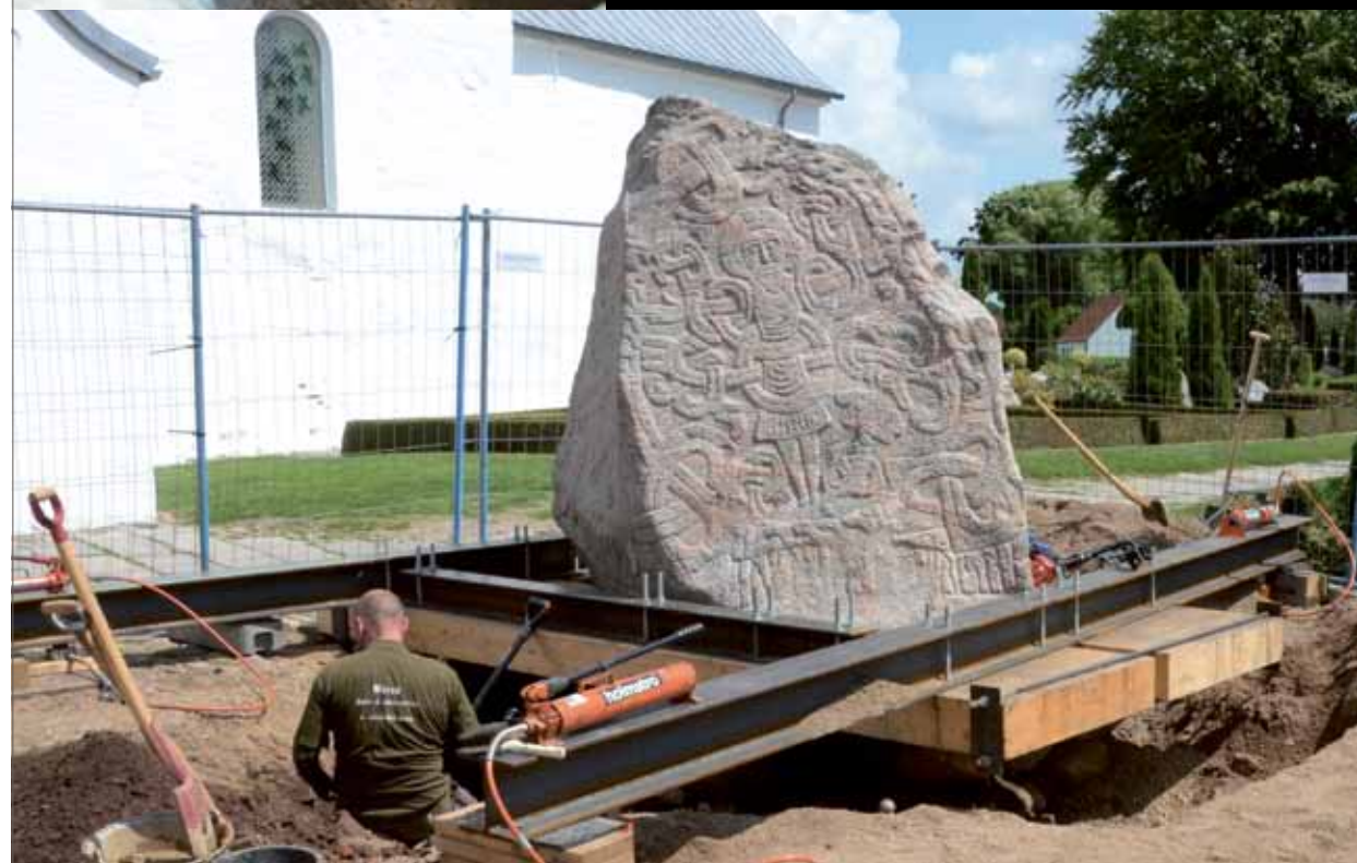
Fig 69 / In May 2011, temporary support for the large rune stone is established.
